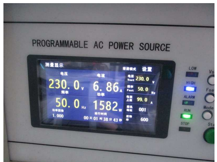
Power test: ok
